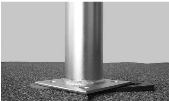
In combination, shims ( \frac{1}{16} " and tapered) level standoff.
