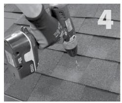
Using drill with 7/32" bit, drill pilot hole into roof and rafter, taking care to drill square to the roof. Do not use mount as a drill guide.
