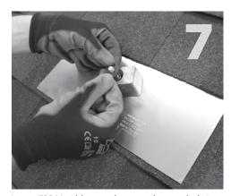
Insert EPDM rubber washer over hanger bolt into block.
