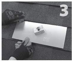
Slide mount into desired position. Remove any nails that prevent getting the mount flush with front edge of shingle course. Mark center for drilling.
