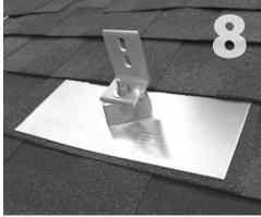
Using the rack kit hardware, secure the rack of your choice. Tighten to 13 foot pounds.
