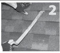
Carefully lift composition roof shingle with roofing bar, just above placement of Quick Mount.
