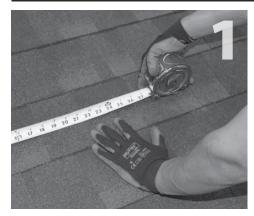
Locate, choose, and mark centers of rafters to be mounted. Select the courses of roofing where Quick Mounts will be placed.
