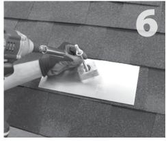
Slide mount back into position. Prepare hanger bolt with 1 hex nut and 1 sealing washer, insert through block into hole and drive hanger bolt into rafter, tightening to a solid snug fit. \*
