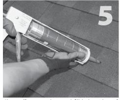
Clean off any sawdust, and fill hole with roof manufacturer's approved sealant.
