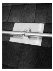
**2. DRILL PILOT HOLE** Using a drill with a 3/16" long bit, drill pilot hole through roof and rafter, taking care to drill square to the roof.
