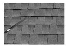
**3. LIFT COMPOSTION** Lift composition roof shingle with roofers bar, just above placement of Conduit Mount.
