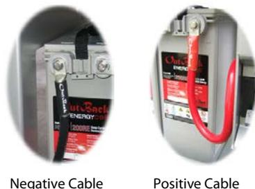
**Figure 6 Battery Connections**
