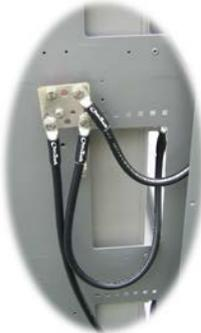
7. Connect a ground cable to the battery rack. The ground terminal is located directly below the negative bus bar (see right). Make sure to follow all applicable electrical codes when grounding the rack.
