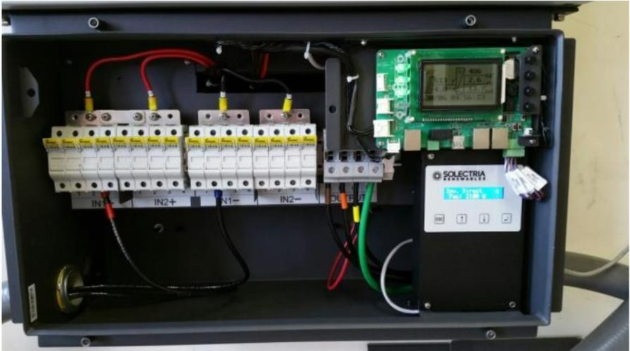
Figure 8.3 – SolrenView Monitoring Installed Inside Wiring Box
